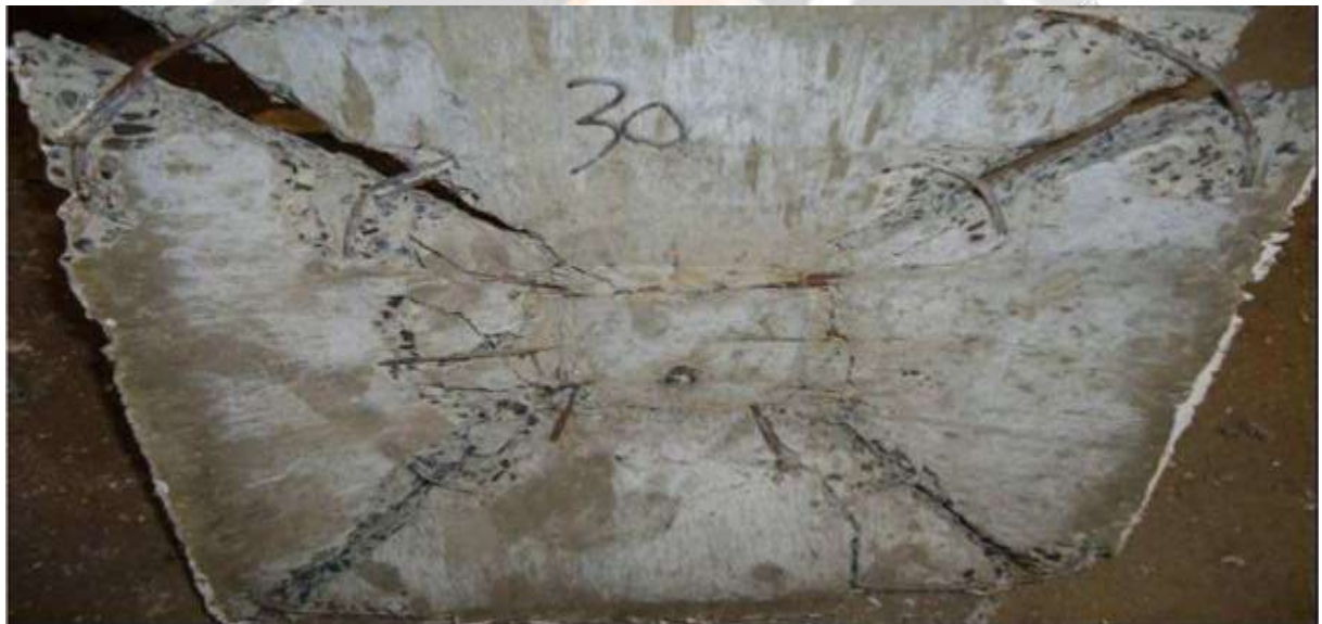
Fig. 4.5 Bottom Failure of 30 degree folded footing during a constant load
