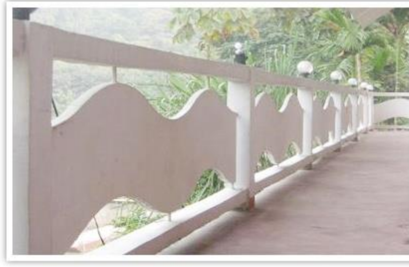
Fig.3 Features of Ferrocement Construction
