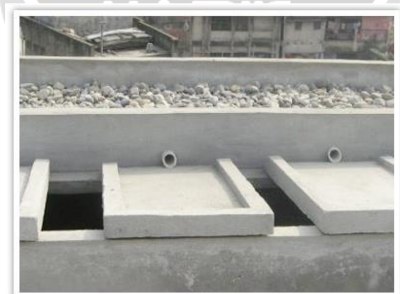
Fig.4 ferrocement formwork
