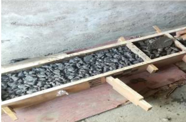
Fig 3: Preparation of Pervious Concrete Prism
