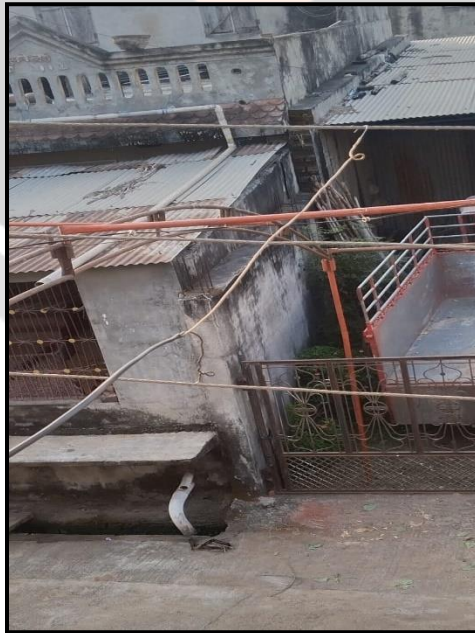
Fig -2 : Illegal Hooking
