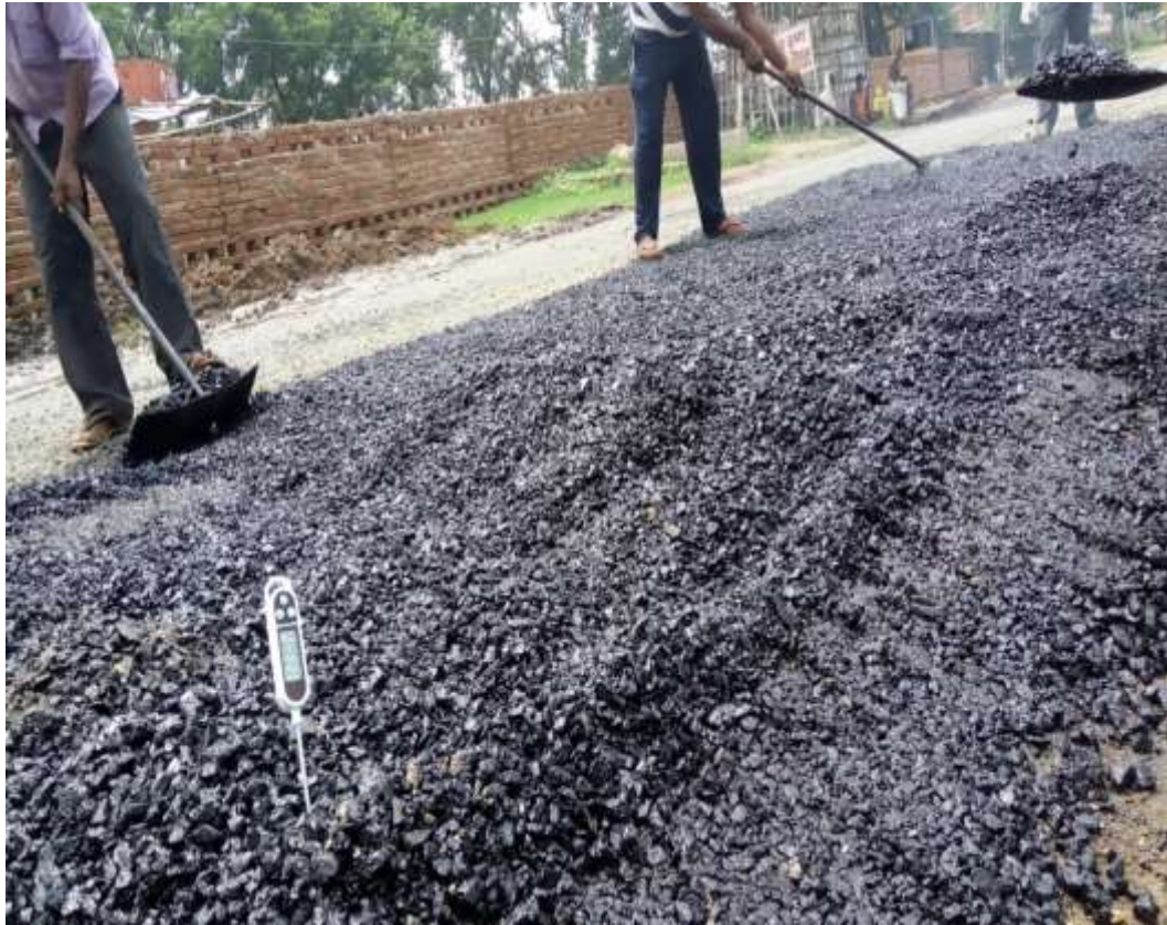
Figure: 6.1 Thermometer used for temperature measuring in bituminous
