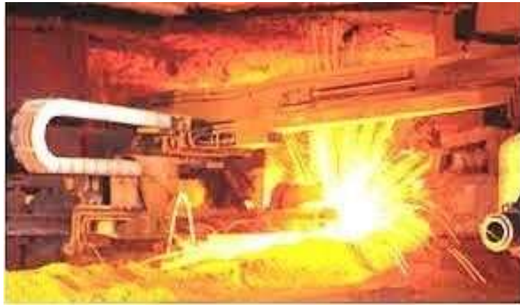
Figure 4 A drilling machine is used to drill the tap hole to tap hot metal from the Furnace
