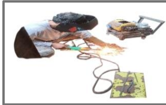
Fig -5: Fabrication of Components
