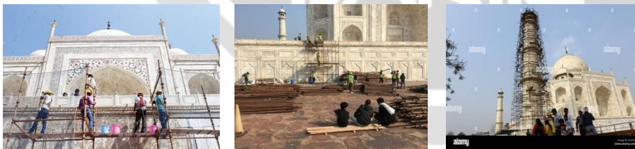
Figure 7 Conservation Project done for Taj Mahal, India
