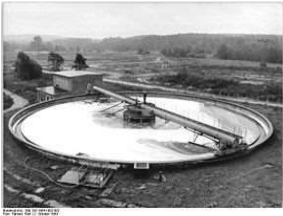
Fig -2: Primary settling tank of wastewater treatment plant in Dresden-Kaditz, Germany
