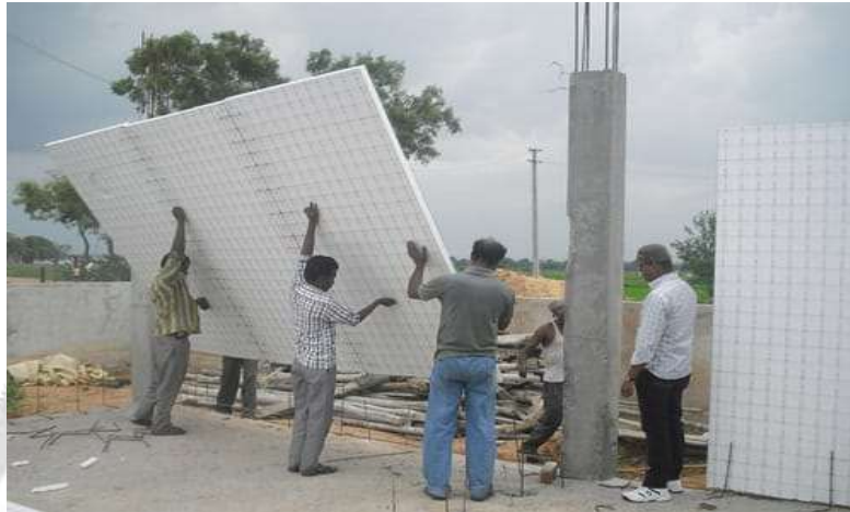
Construction of EPS wall panel
