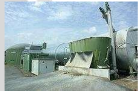
Farmyard anaerobic digester converts waste plant material and manure from livestock into biogas fuel.
