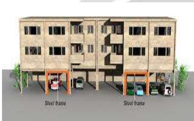
Fig. 1.1: Building with opening at base.
