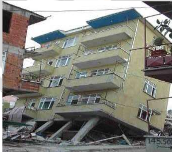
Fig. 1.1: examples of failure of buildings with soft storey at ground floor
