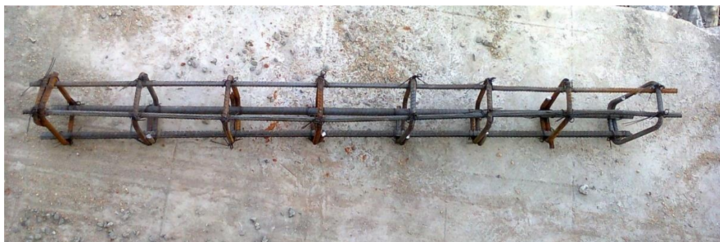
Figure 4.2.4 Beam Reinforcement
