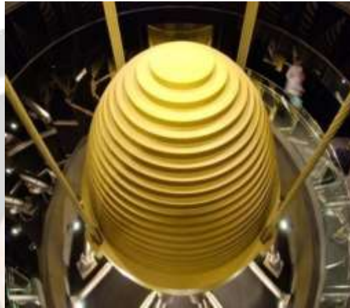
Fig.1.4 Tuned mass Damper
