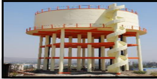
Figure. 1 Concrete water tank.
