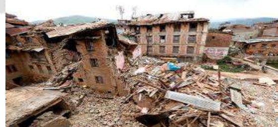
Fig.2 Collapsing of Building
