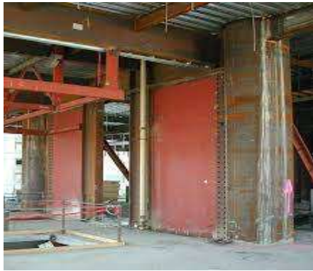
Fig.14 Steel Plate shear wall
