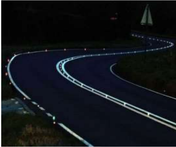
Figure3: Solar Roadways at Night Time on the Curved Road.
