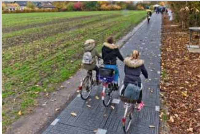
Fig- 3: Solar powered Roads.
