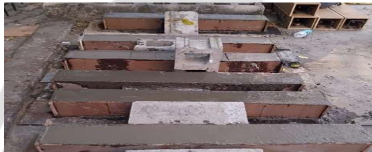
Fig 5.5 Casting of Beam Specimen
