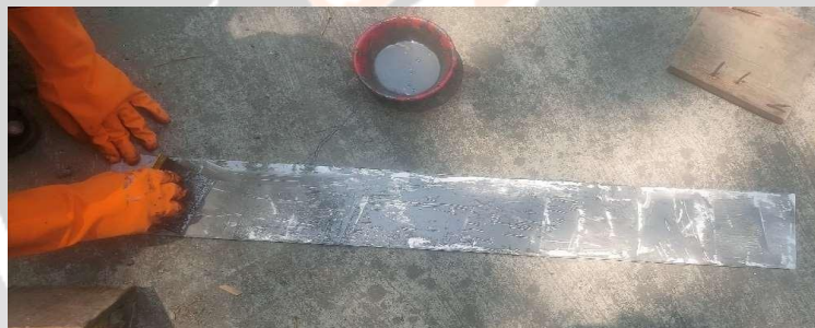
Fig 5.6 Applying Epoxy in Aluminium Alloy Plate
