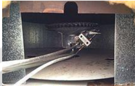
A thermocouple (the right most tube) inside the burner assembly of a water heater.
