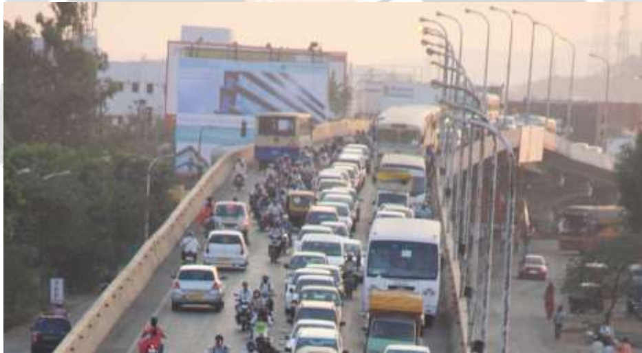
Fig -1: Hinjewadi-wakad flyover
