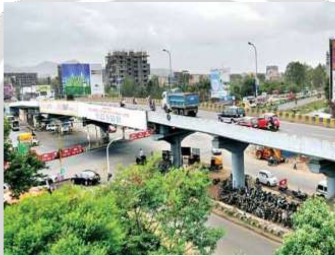
Fig -2: existing structure at Hinjewadi – waked flyover.
