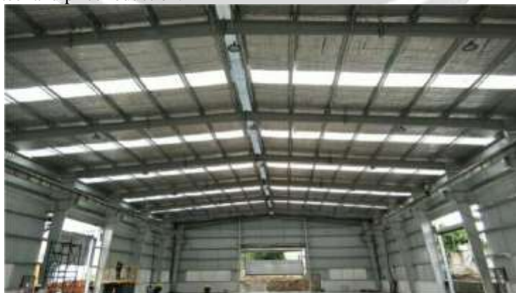
Fig. 1: Pre-Engineered Warehouse Structure
