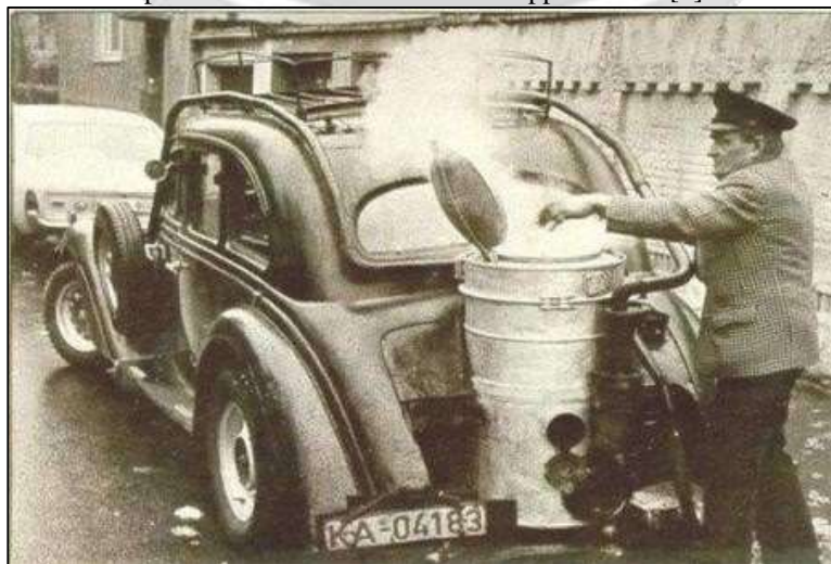
Photograph : Car Powered by Biomass Gasifier during World War-II
